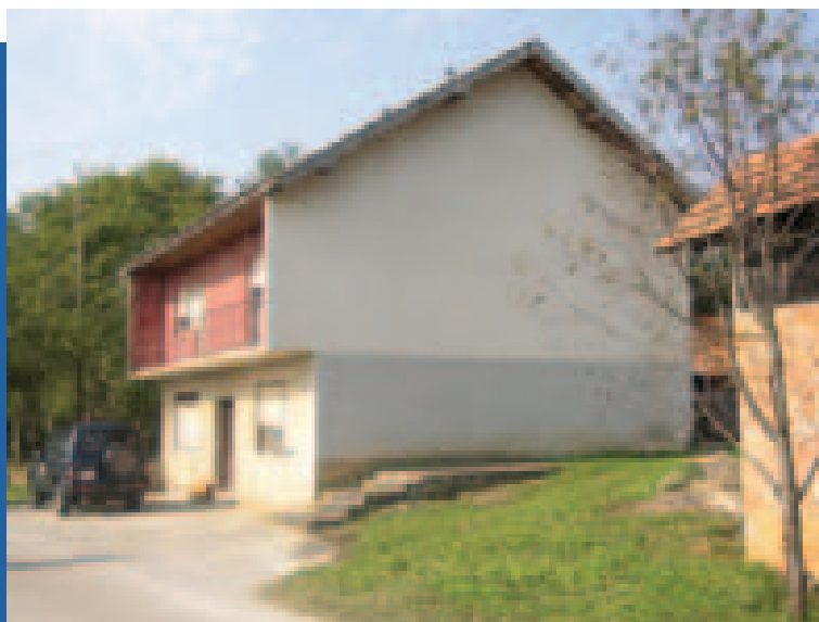
Figure 5. A repossessed house
